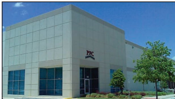
PFC S.W. Regional Distribution Center, Dallas, Texas
